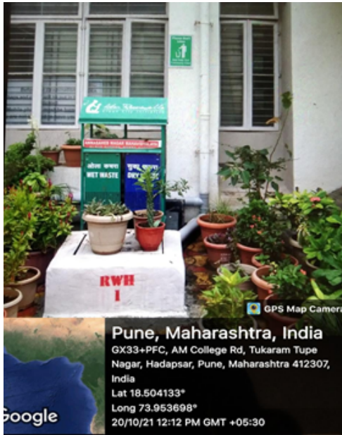
Rain harvesting unit 1
